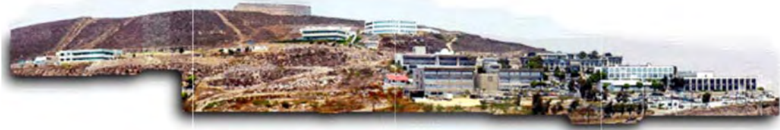
FIGURE 18. CICESE's present facilities.
