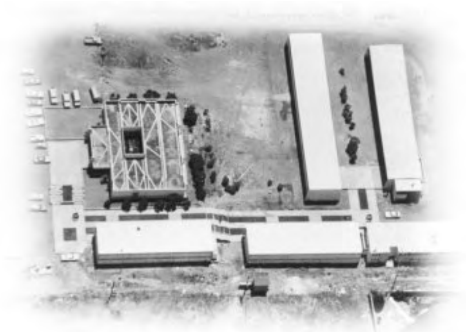
FIGURE 9. The Escuela Superior de Ciencias Marinas under construction, in 1974 (aerial view).
