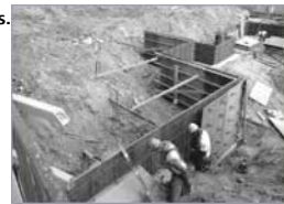
Laying the foundations for the new IGPP Revelle Laboratory
