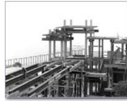
Construction of Revelle Lab Building 4000 and the Scripps Crossing bridge
