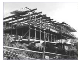
Construction of Revelle Lab Building 2000
